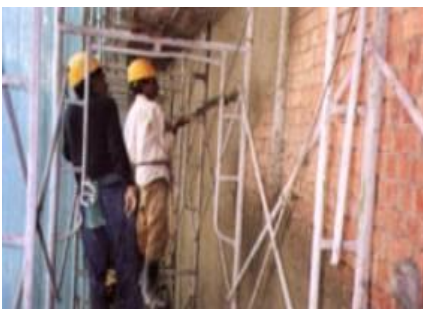
Spraying Mortar
